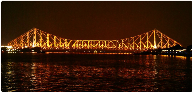
The iconic steel cantilevered Howrah Bridge illuminated over the Hooghly River.
